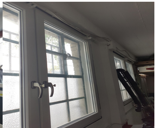
↑ New soundproof and lockable windows.
